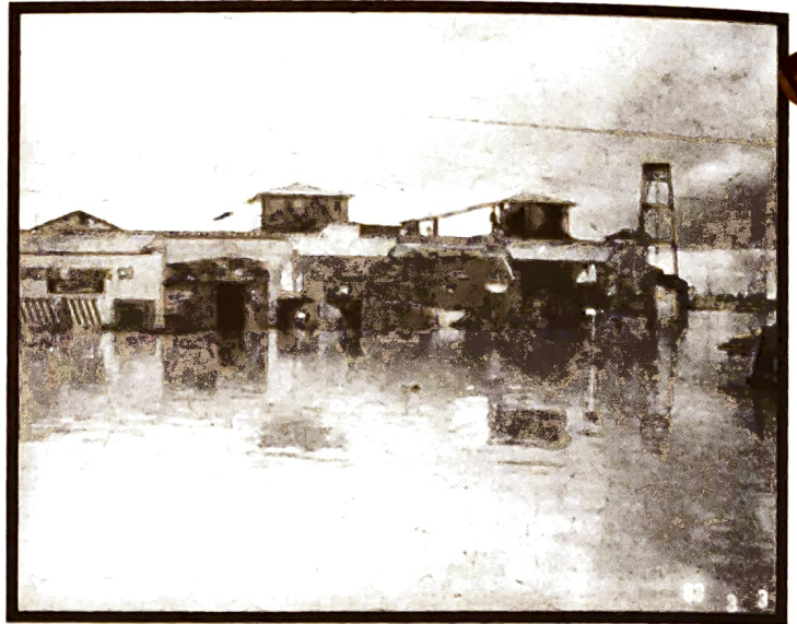
The historic Bayside Canning Company building (home of the San Francisco Bay Bird Observatory) appears to float on seven foot deep flood waters after torrential rains in March 1983. Photo courtesy of the Santa Clara Valley Water District.
